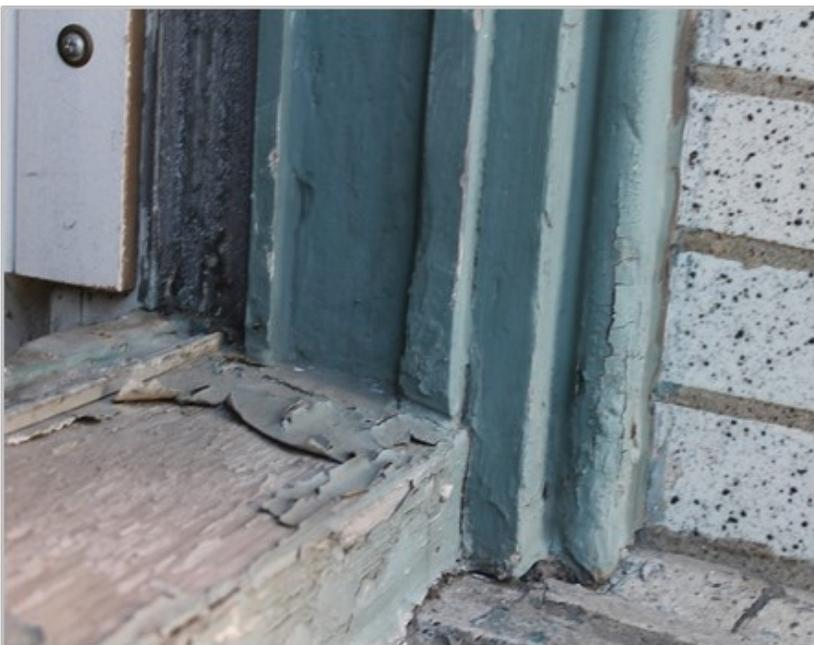
4. Wood Double-Hung—Sill, Jamb, Brick Mould, Parting Bead and Stop Bead,
